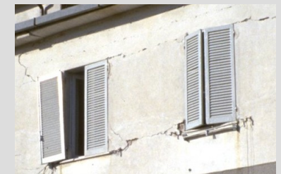
Rocking failure
