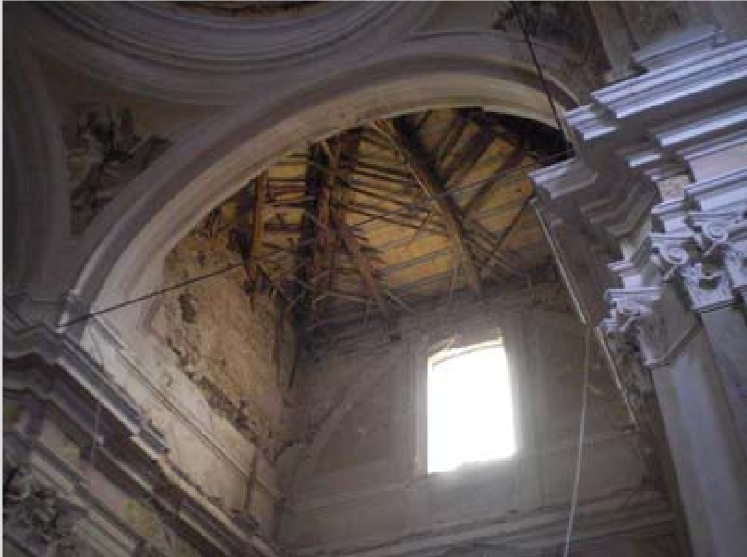
New r.c. roof in the transept (1960/70) (all other roofs are in timber and the only vault that collapsed is in the transept)
