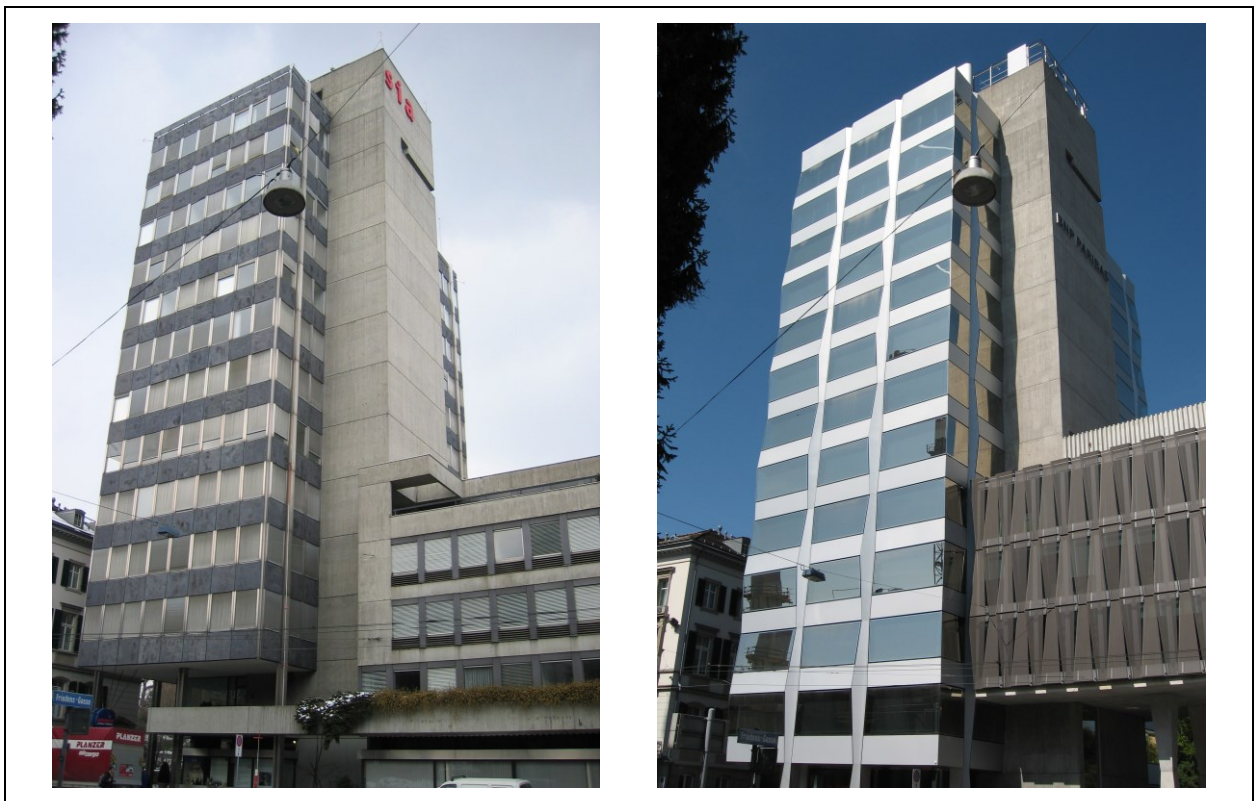
Figure 1.2: Example for the assessment and retrofitting of an existing building [05]
