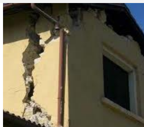
Mechanism 2. Kinematic failure mechanism - out-of-plane seismic actions
