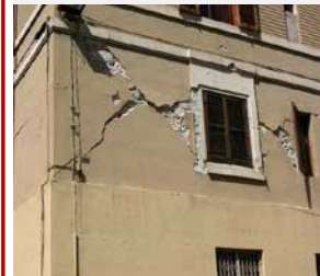
Mechanism 3. Kinematic failure mechanism in-plane
